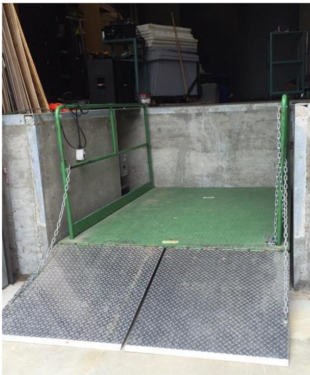
Lift lowered for ground level load-in & interior view. Railings are removeable.
